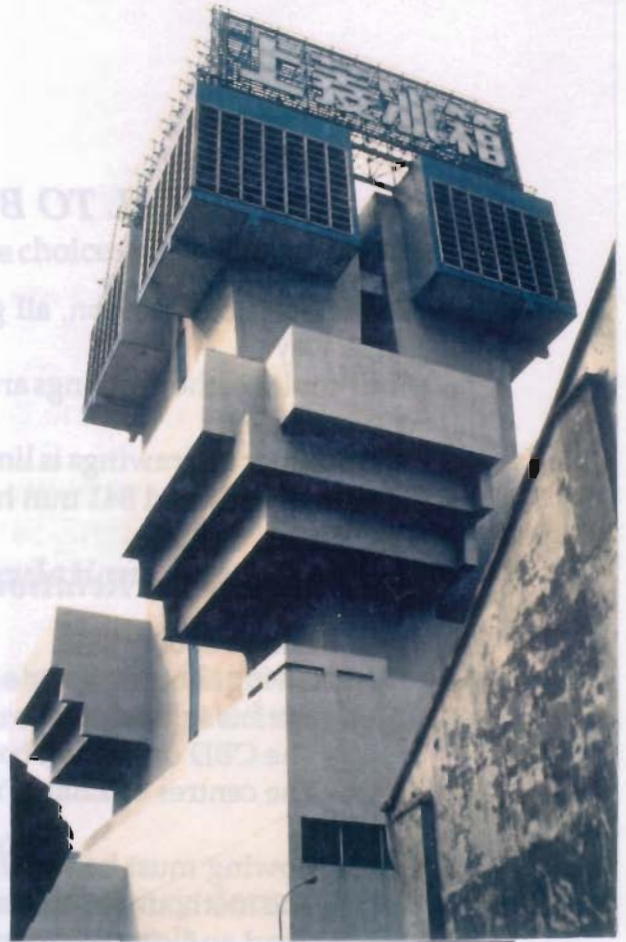
Tunnel ventilation tower
